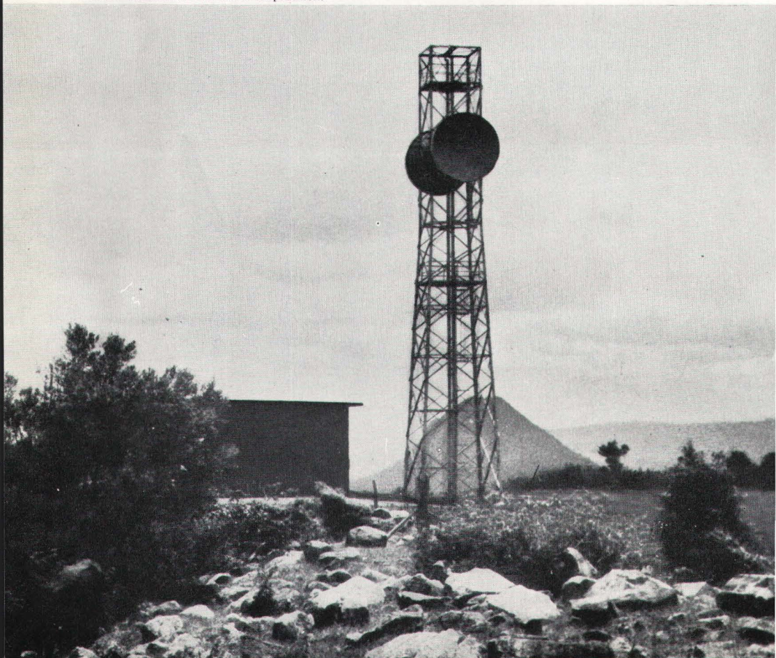
COMMUNICATION—Chapter 8 Brisbane-Cairns microwave radio link repeater station at Black Mountain, near Cooroy
